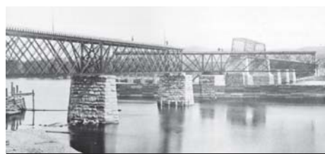
Swing bridge in the open position. Note the balancing beam at the bottom of the swing section.
